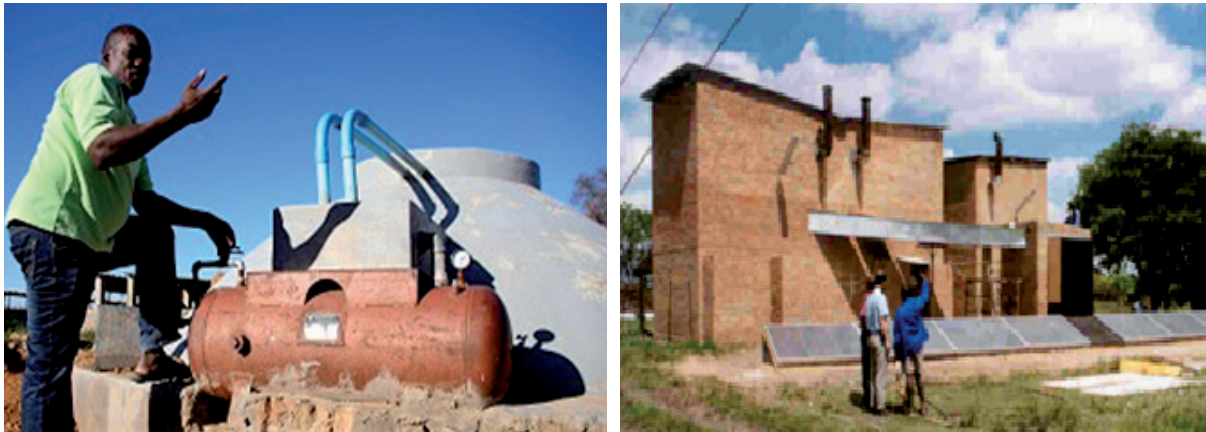
Figure 11.5 Use of biogas digester at Victory Farm (Beatrice) and solar application in tobacco barns
